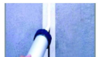
Step 2: Fill the gap with VIVA Flex
